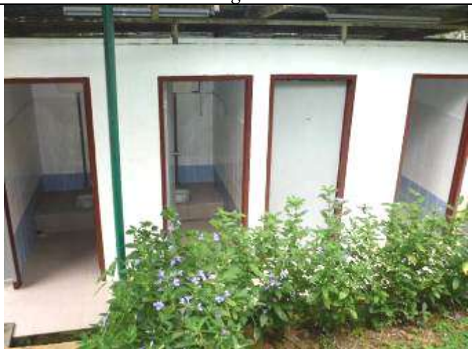
Outside toilet (4 units)
